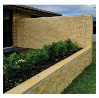
Split BayRidge® used in a feature wall and garden bed design with smooth capping.
