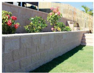
Split BayRidge® used in as a retaining wall with smooth capping.
