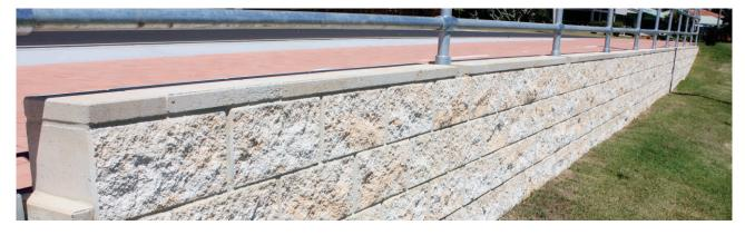
Split BayRidge® used in as a retaining wall with smooth capping.
